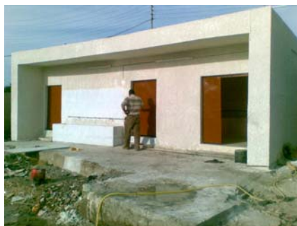
Batool school's toilets rehabilitated. Photo: UNICEF
